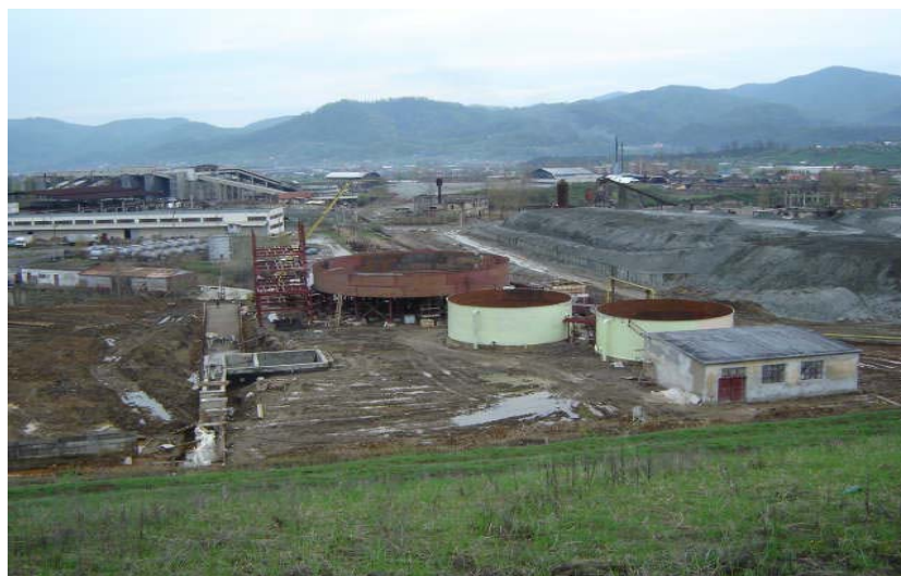
Overview of Central Tailings Slurry Plant Site
